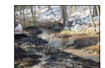
Create a channel with a connection to its floodplain. Incorporate meanders to promote dissipation of energy.
